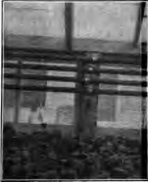
14.—Fastening pipes to posts by tin clips.
